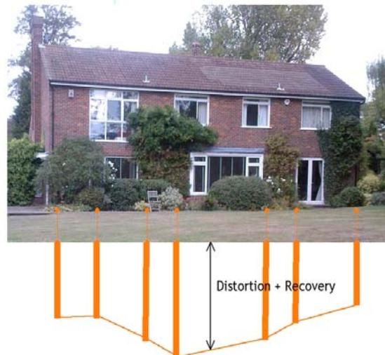
A variety of trees and shrubs exist within influencing distance of the damaged building and the study compares a range of soil tests (oedometer, suctions, moistures, penetrometers etc) with results obtained from a precise level survey with some interesting results.
